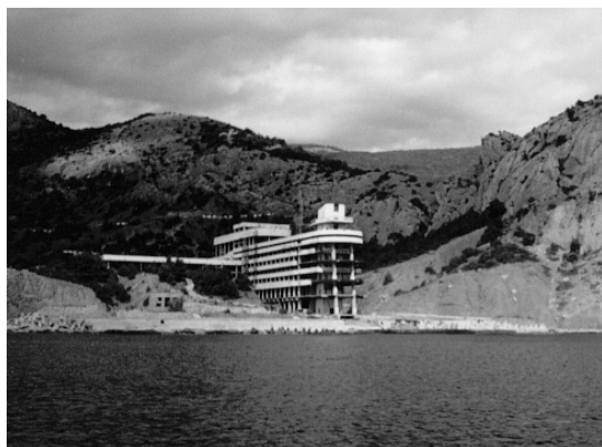
Figure 7. The coastal area of the "Dolphin" Sanatorium, Sudak
